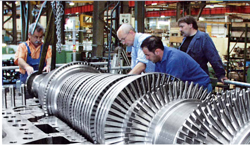
Fitting of rotor into the casing of the new MARC 4-B10 steam turbine for the Hagenholz Plant.
