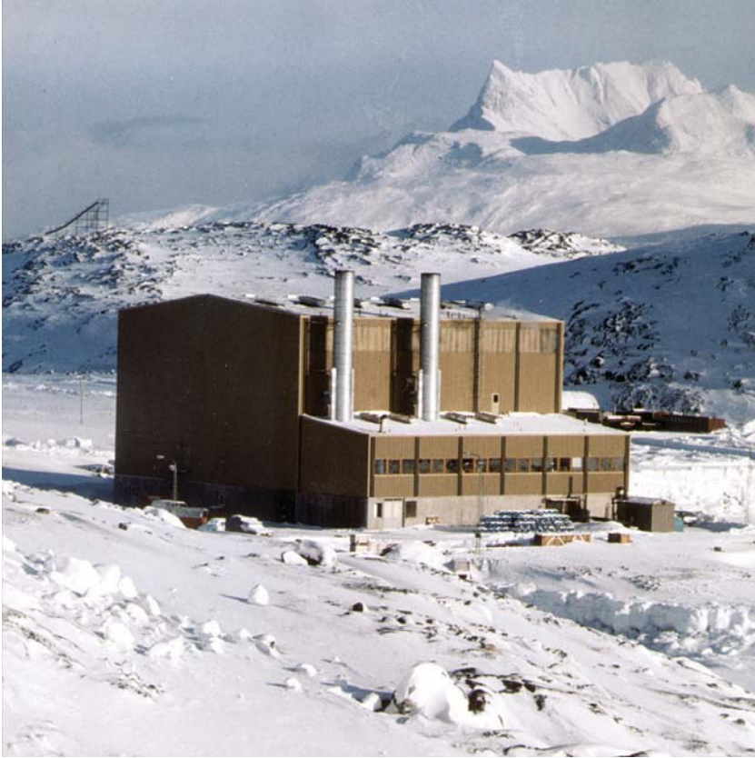
13 MW power plant at Nuuk, Greenland
