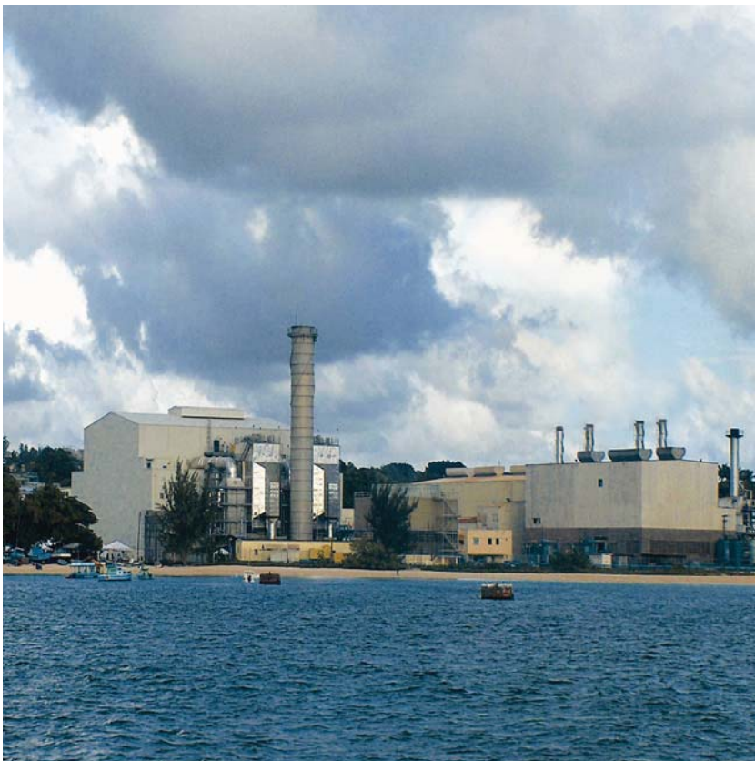
60 MW BLPC, Barbados 2 x MAN B&W 9K80MC-S, Electrostatic Precipitator
