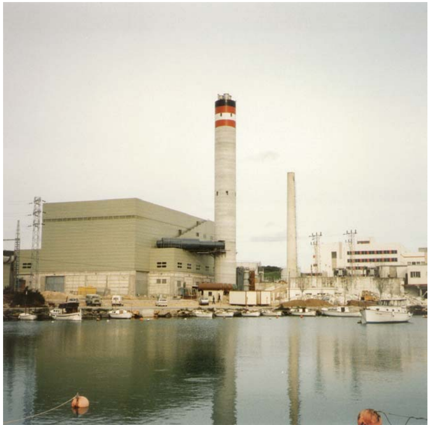
48 MW power plant at Menorca, Spain
