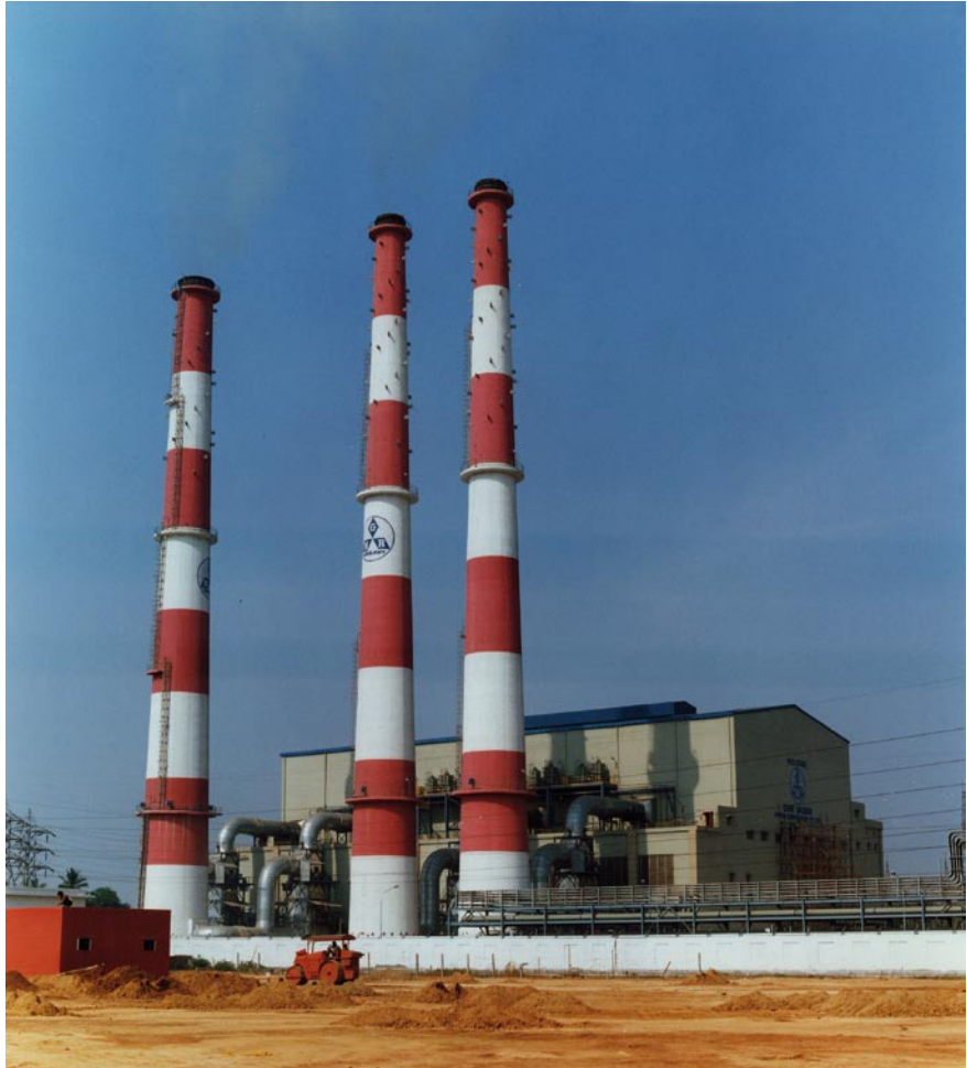
Fig. 19: 200MW GMR plant at Chennai Power
